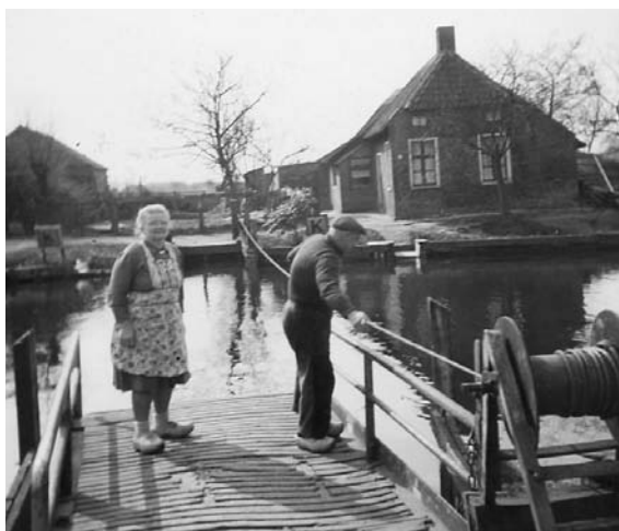
| De pont in Belt-Schutsloot
